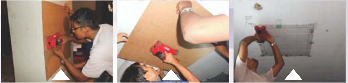
Rebar Scanning Using Ferro Scan in Column, Beam & Slab respectively
