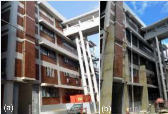
Building (a) before and (b) after retrofitting
